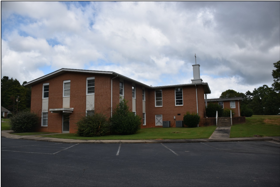
Figure 2.1.14. Oblique of education annex, West Bend United Methodist Church, facing northeast.
