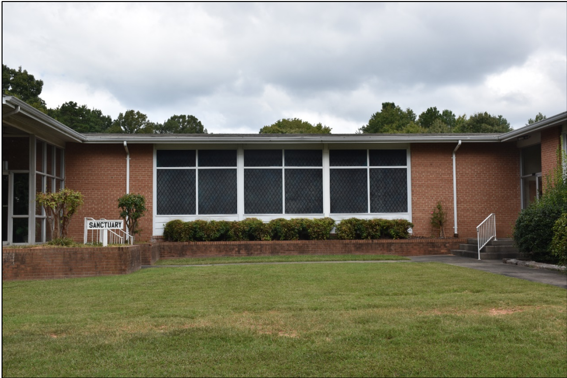
Figure 2.1.11. Front elevation of central hyphen, West Bend United Methodist Church, facing north.
