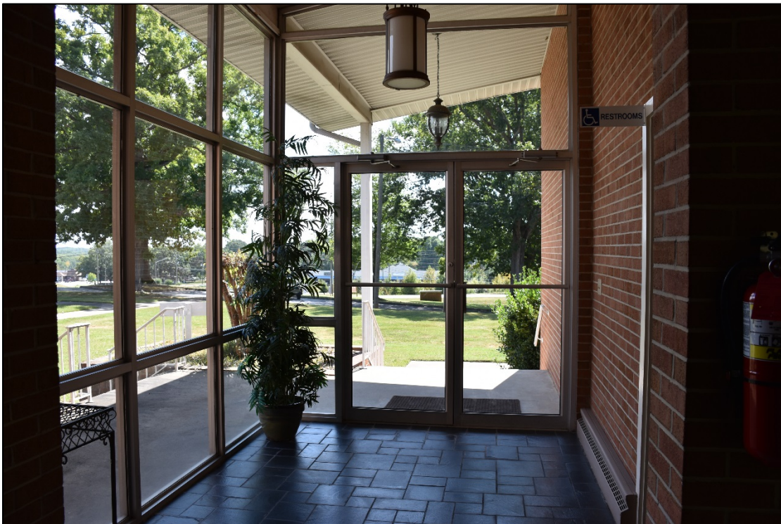
Figure 2.1.24. Glass vestibule, west wing, West Bend United Methodist Church, facing south.
