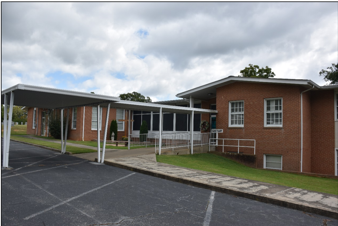
Figure 2.1.10. Rear oblique of western wing, West Bend United Methodist Church, facing southeast.
