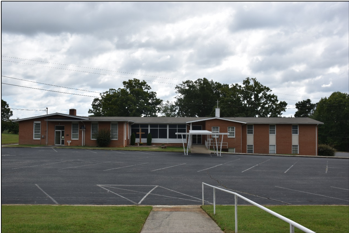
Figure 2.1.12. Rear elevation, West Bend United Methodist Church, facing south.
