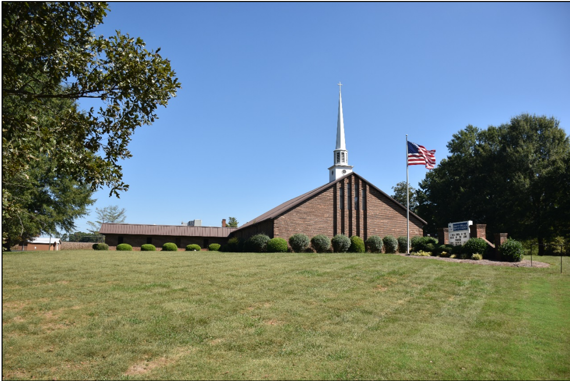
Figure 2.1.33. Amity Hills Baptist Church, facing northeast.
