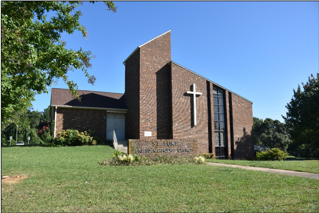
Figure 2.1.34. St. Luke United Methodist Church (RD0393) (1971), facing north.
