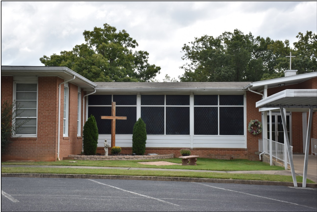
Figure 2.1.13. Rear elevation of central hyphen, West Bend United Methodist Church, facing south.
