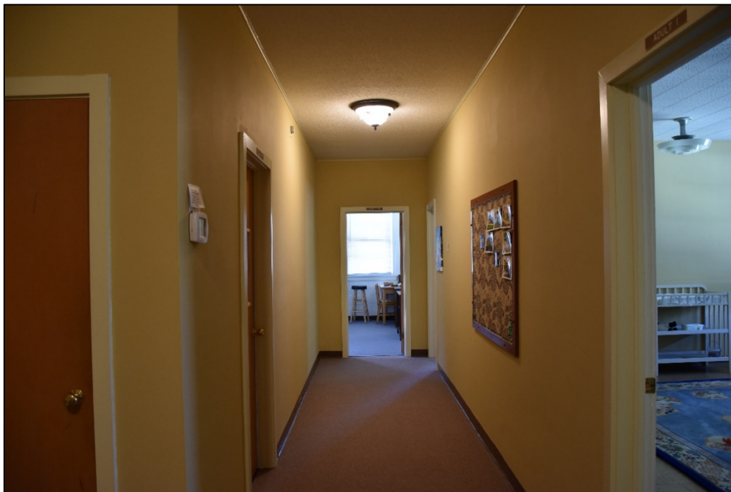
Figure 2.1.27. Classroom wing, upper story of education annex, West Bend United Methodist Church, facing west.
