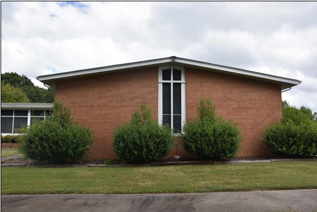
Figure 2.1.4. Front elevation of eastern wing, West Bend United Methodist Church, facing north.
