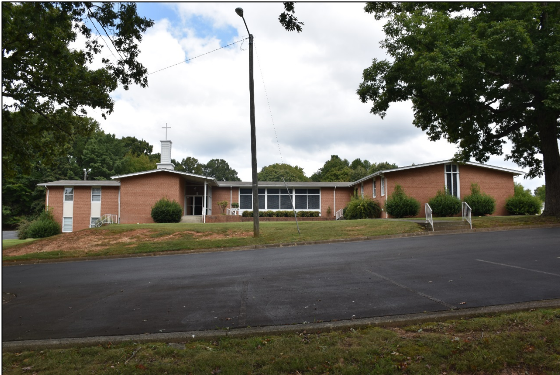
Figure 2.1.1. View of the West Bend United Methodist Church, facing north.
