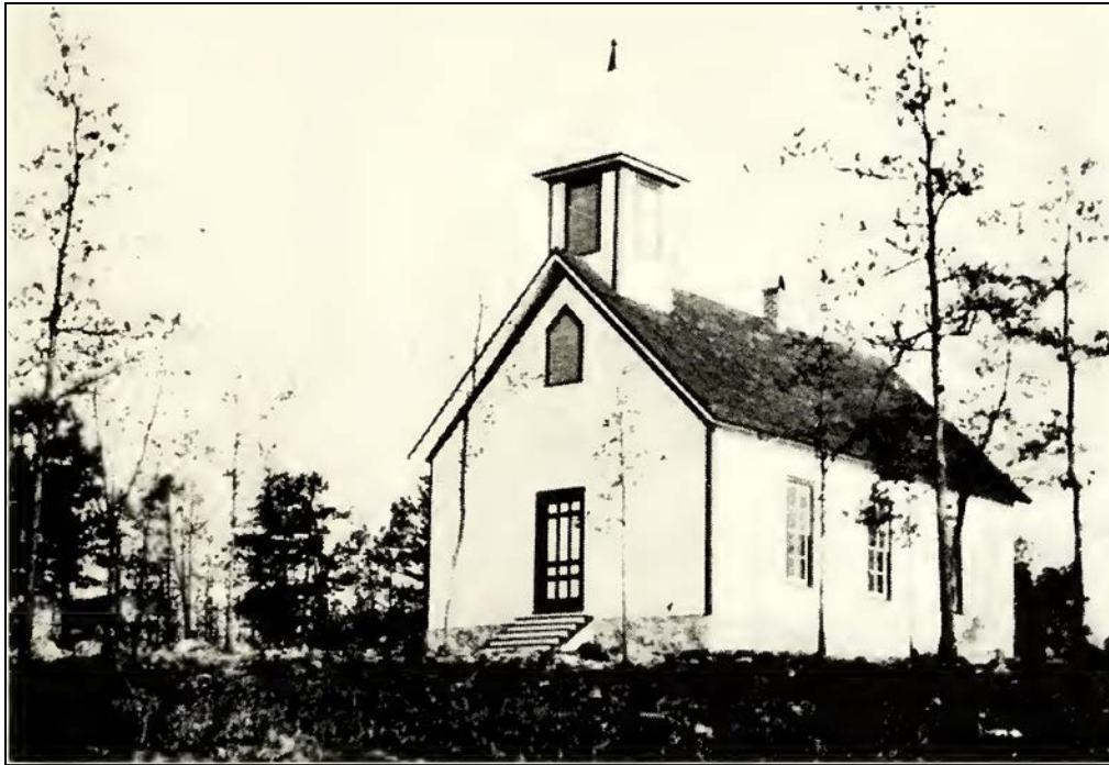
Figure 2.1.29. Photo of West Bend United Methodist Church, 1910 building.
