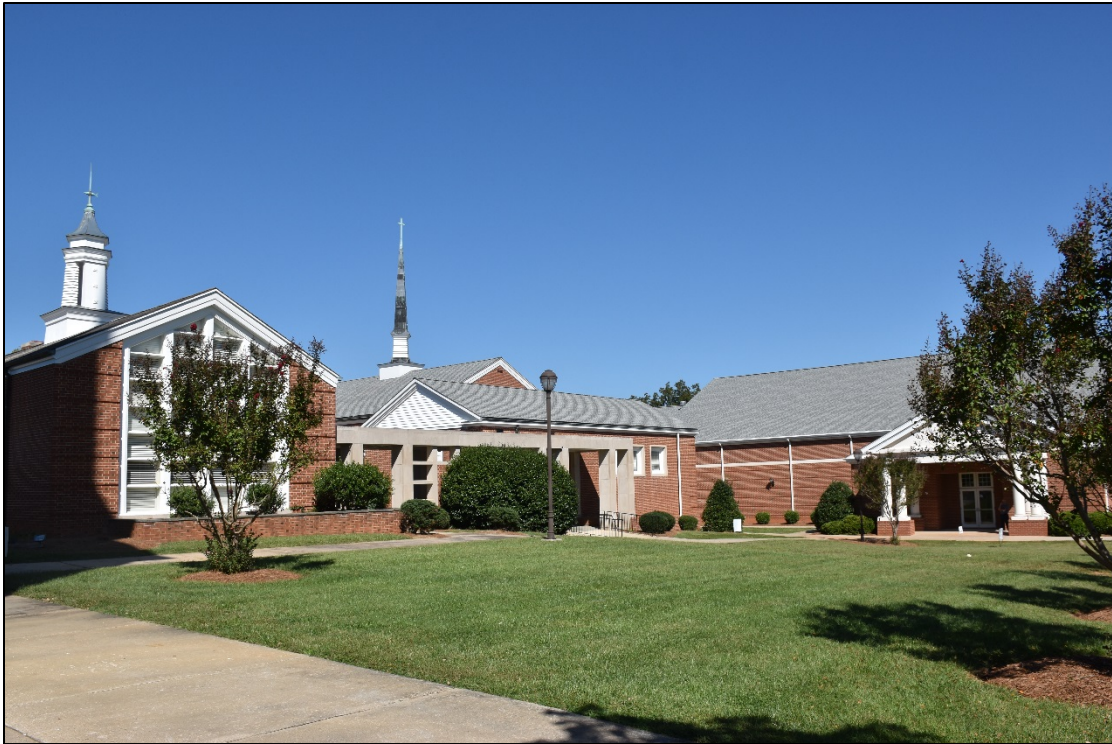
Figure 2.1.36. Central United Methodist Church (RD0503) (1968), facing northwest.
