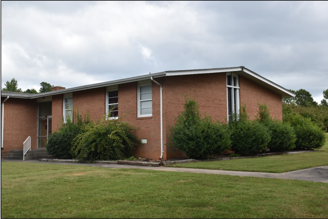
Figure 2.1.5. West elevation of eastern wing, West Bend United Methodist Church, facing northeast.
