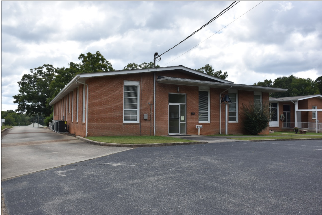
Figure 2.1.7. Rear oblique of eastern wing, West Bend United Methodist Church, facing southwest.
